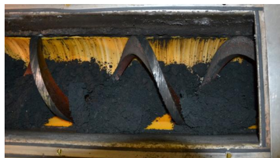
Fig.2, Screw conveyor for transporting sewage sludge and HTC coal into the oven of the sewage sludge incineration plant (SVA)
